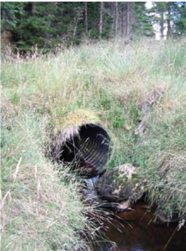
*A forestry road culvert on the Glenmulliach Burn prior to removal. This type of river crossing is commonplace in Scotland (and Scandanavia) and can cause extensive problems for fish access. Electro-fishing surveys confirmed that this particular example prevented upstream access for trout due to the height the pipe was placed above the water level.*
