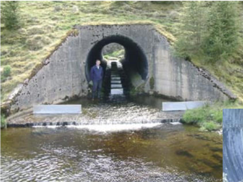
*Graeme Dunlop (Moray Council) inspects the newly installed baffles on the Blair na Marrow culvert.*
