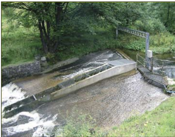
Mortlach weir with Denil fish pass completed. The VAKI counter is housed in the upper chamber of the fish pass.
