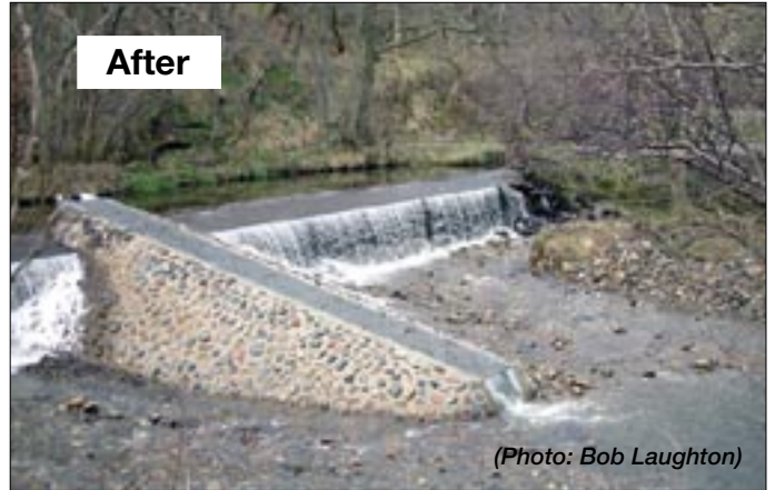
Dufftown Distillery weir: In partnership with Diageo, a new Denil fish pass has been installed on the weir to allow fish passage into the Dullan Water.
