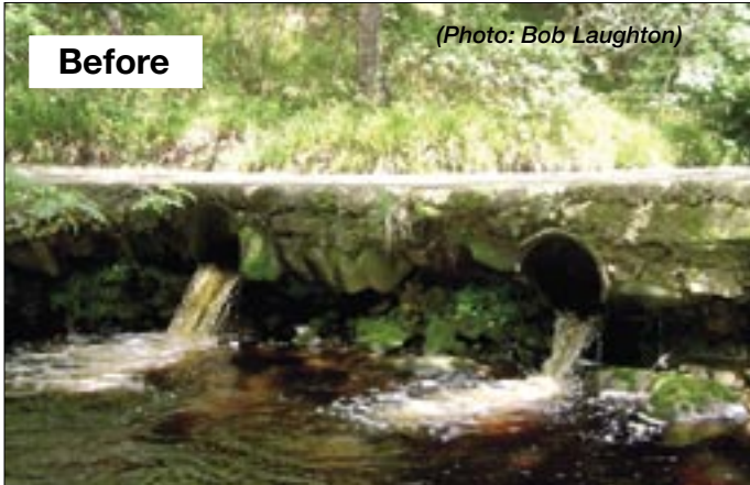
Ballintomb Burn bridge: In partnership with Mr. Chris Martin and the Carron and Laggan Fishings, this impassable culvert bridge has been replaced with a full-span bridge to allow fish passage up the Ballintomb Burn.
