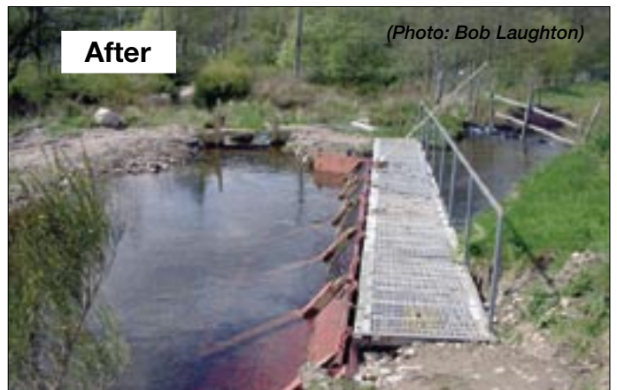
Rothiemurchus Trout Farm screens: Smolt screens have been installed by Rothiemurchus Estate to prevent the loss of salmon smolts and kelts into the trout farm.
