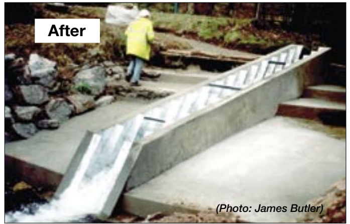
Fochabers Burn fish passes: In partnership with the Crown Estate, two Denil fish passes have been installed on weirs at the downstream extremity of the Fochabers Burn
